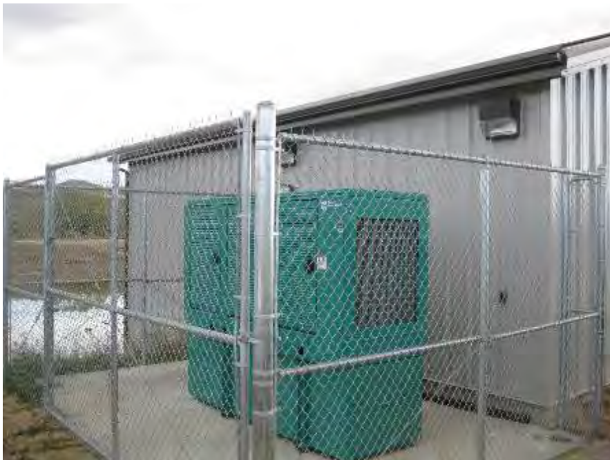
BPSOU: backup power generator next to D4
