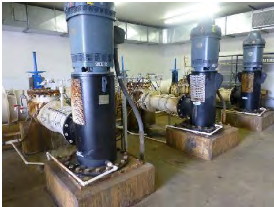
Warm Springs Ponds: Water level pumps
