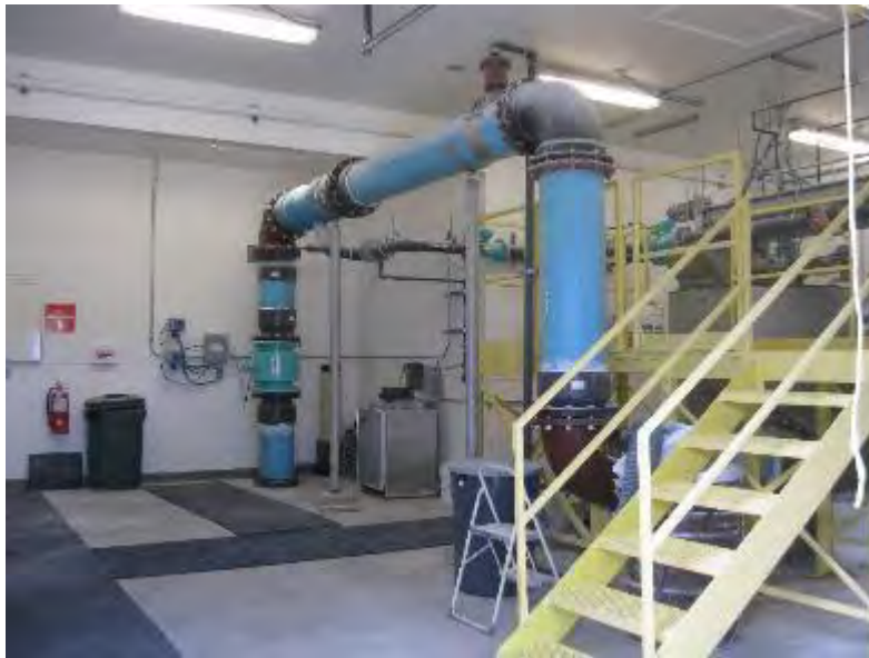
BPSOU: Butte Treatment Lagoons Chemical Addition Building – everything is new except stairs and platform
