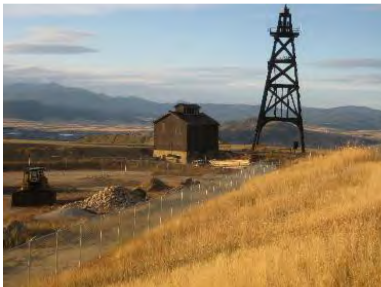
BPSOU: Mining head frame
