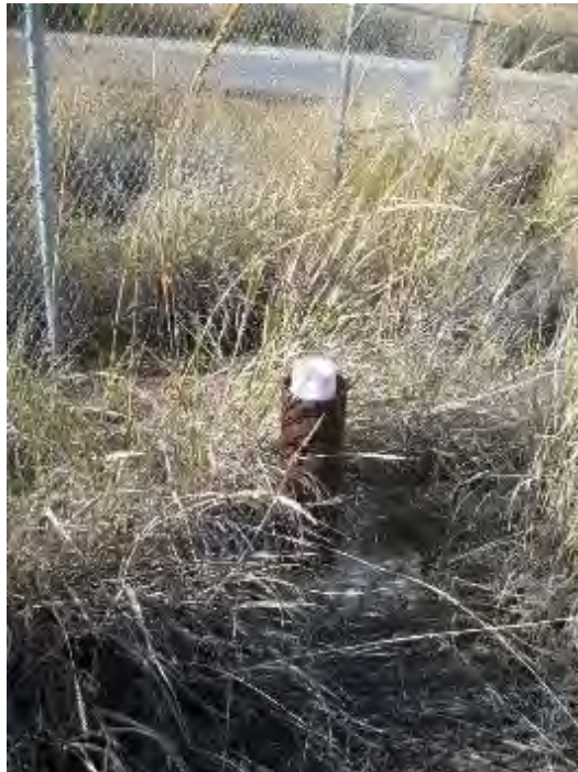
Rocker well with frost heave
