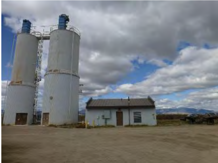
Warm Springs Ponds: Lime treatment silos
