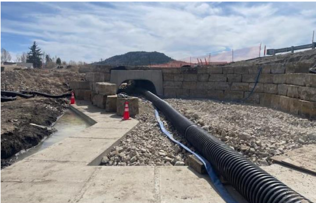
Setting rock block on the north side of the arch culvert. Looking south
